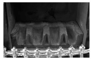
b) Position the two halves of the front ceramic (L/H & R/H) on the locating channel in the front ceramic, ensuring it is located onto the lip on the burner front ceramic support. (See fig. 14 below)
