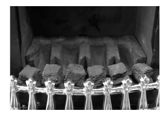
d) Select four of the large coals and arrange behind the front row of coals, ensuring that flame paths as indicated below are not interupted.
